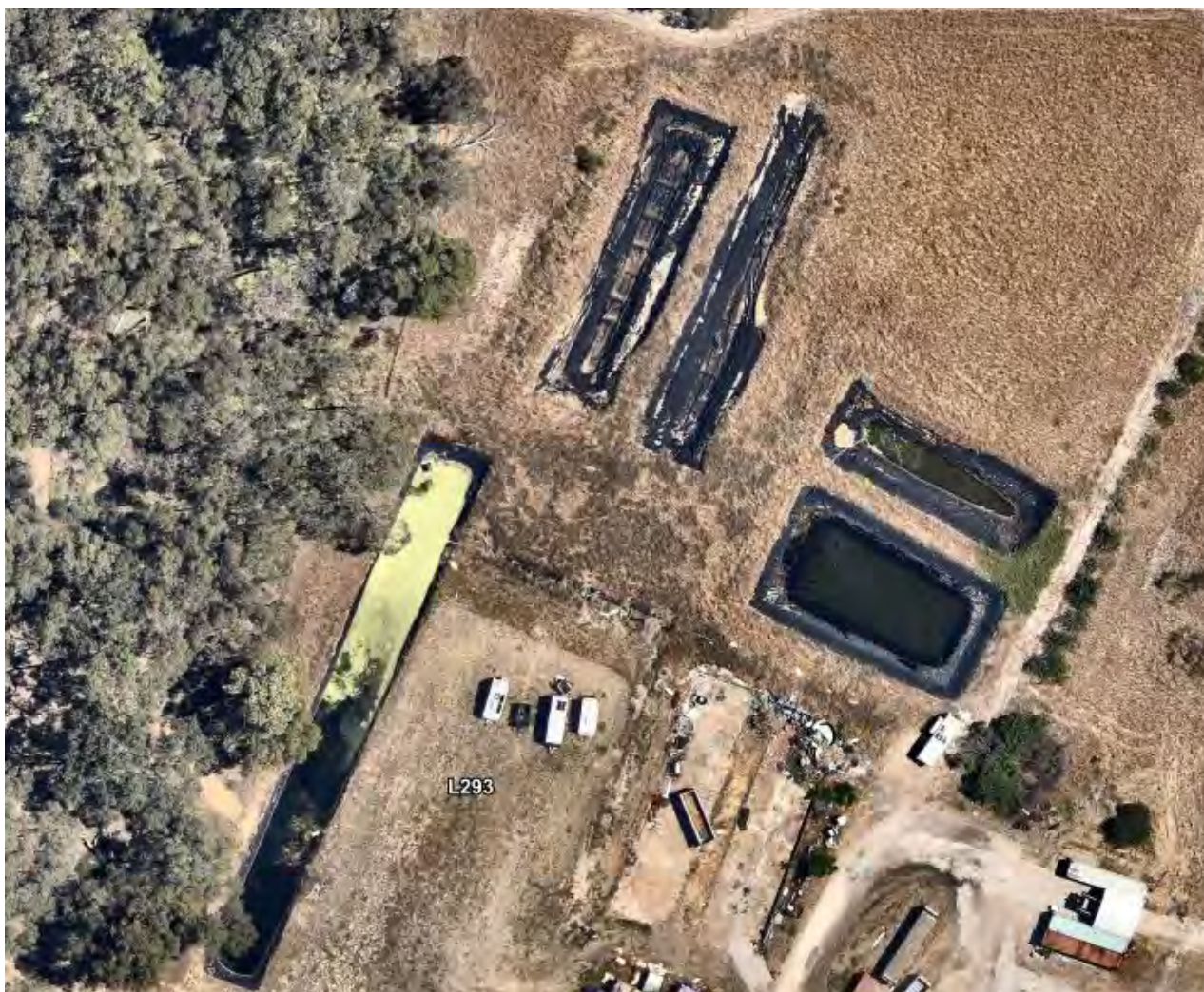
Plate 2-8: Surface water storage areas within Lot 293
