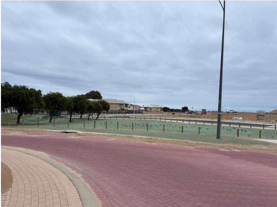
9. Photograph depicting the re-alignment of Long Beach Rise
