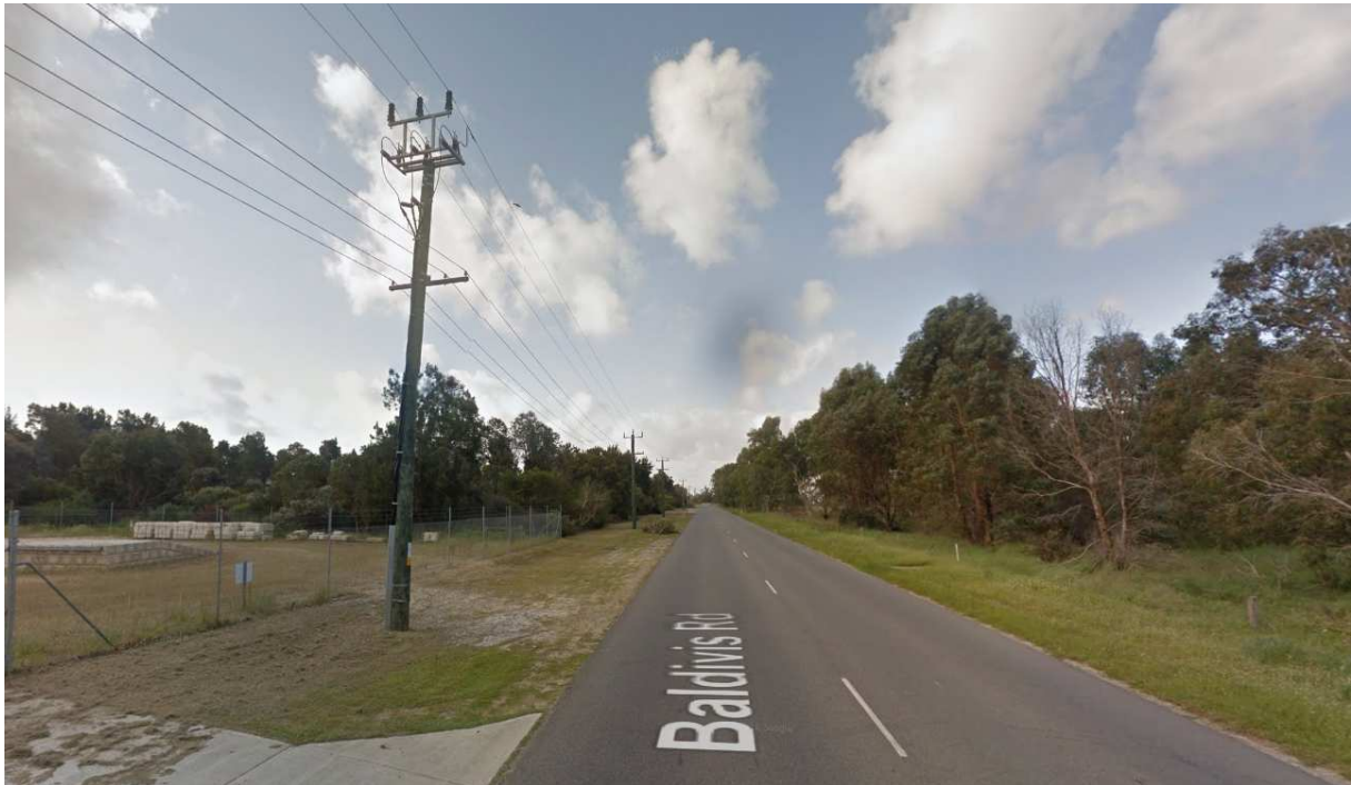
Figure 12 - Looking North from the Proposed Access Point
