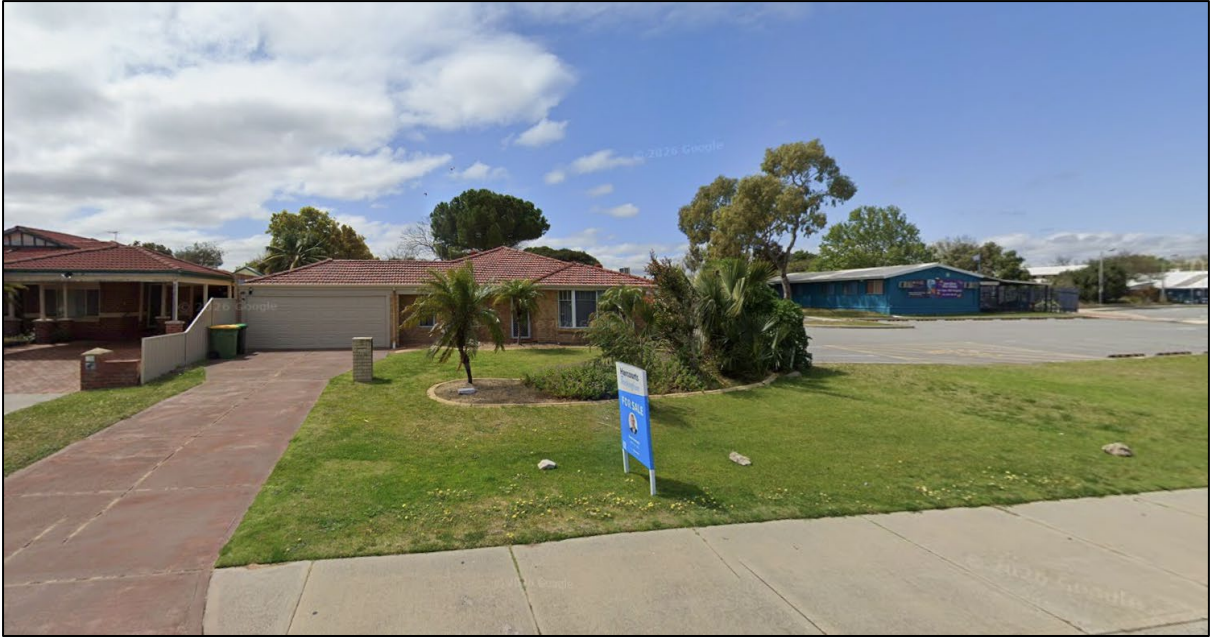
Figure 3: Streetscape Photo – Subject Site
