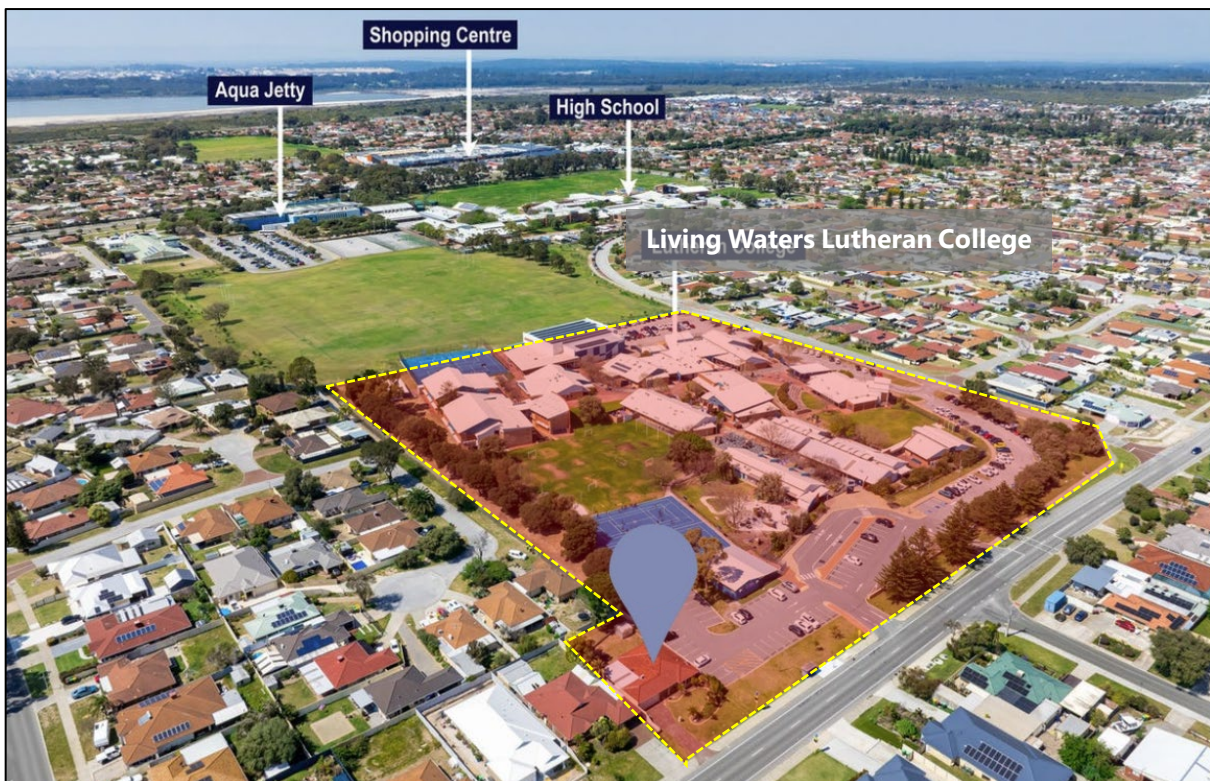
Figure 2: Local Context Aerial - East
