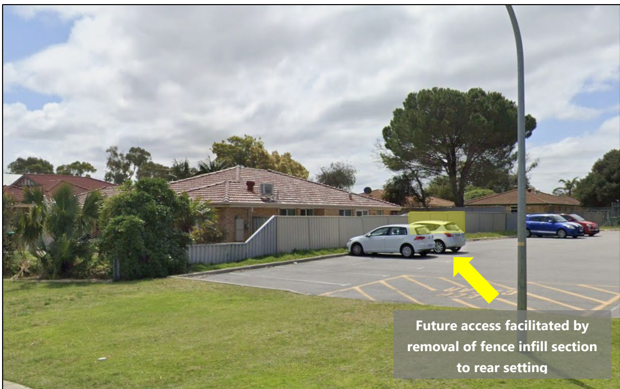
Figure 4: Streetscape Photo – Subject Site view from future access point
