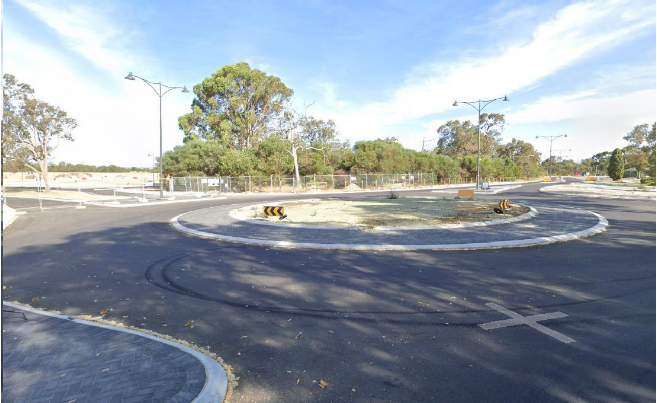
Figure 11 View from Baldivis Road, adjacent to Solis Bvd facing South-East towards proposed site
